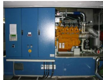
CHP of 330 kWel in Evangelisches Krankenhaus Hubertus Hospital in Berlin, Germany (source: Code2)
